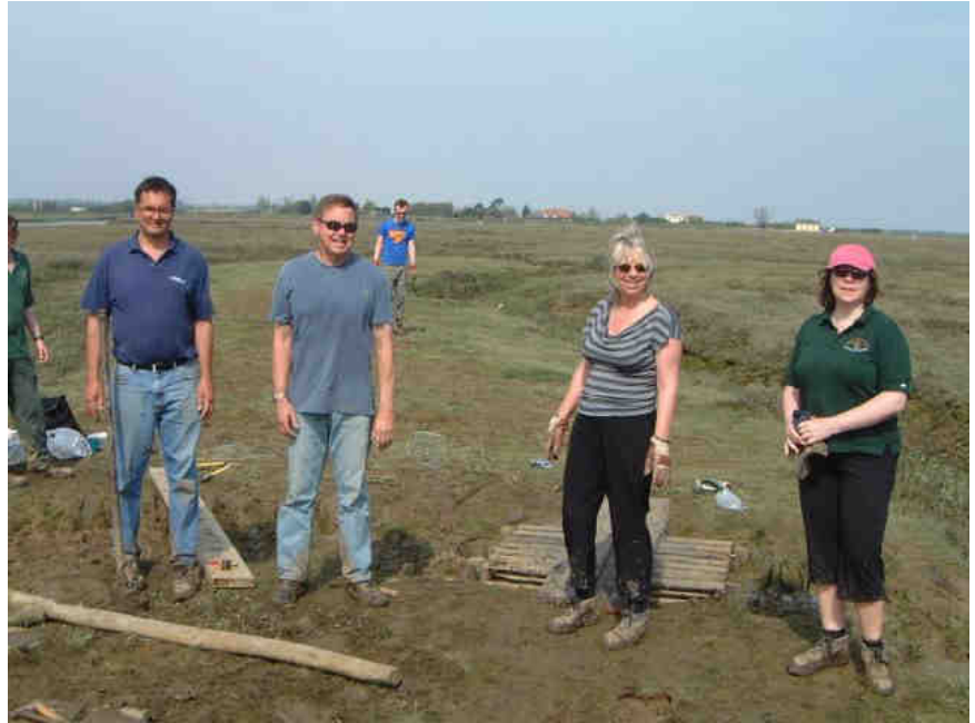
Bridge Building on Ray Island
